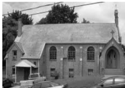
South side of church with main entrance
